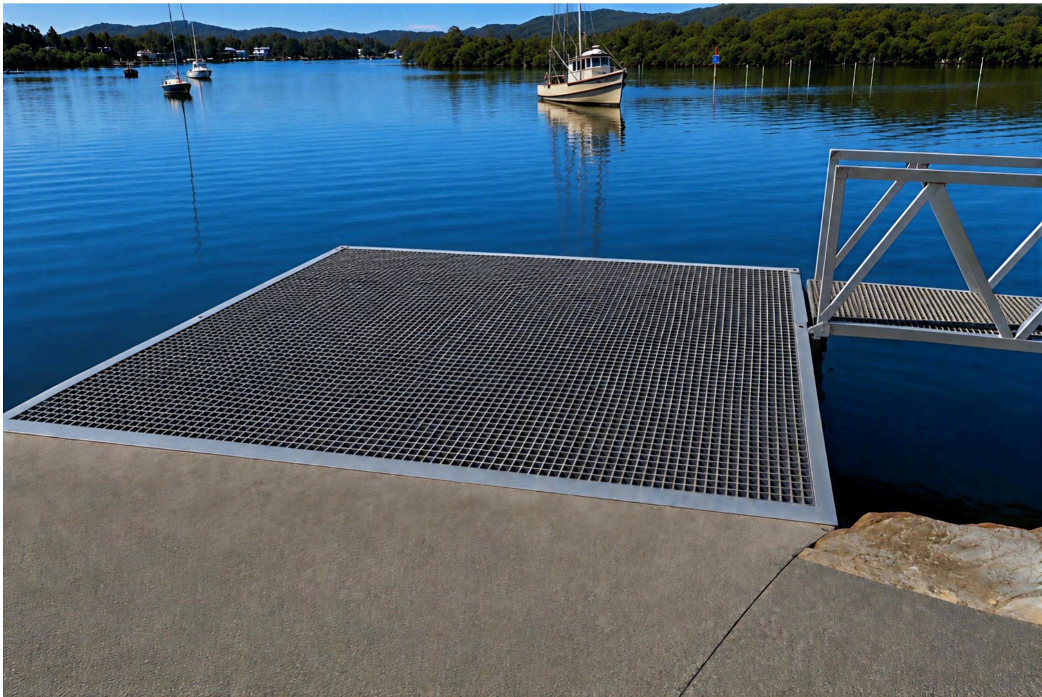
RENEW EXISTING FIXED DECK WITH LARGER DECK
