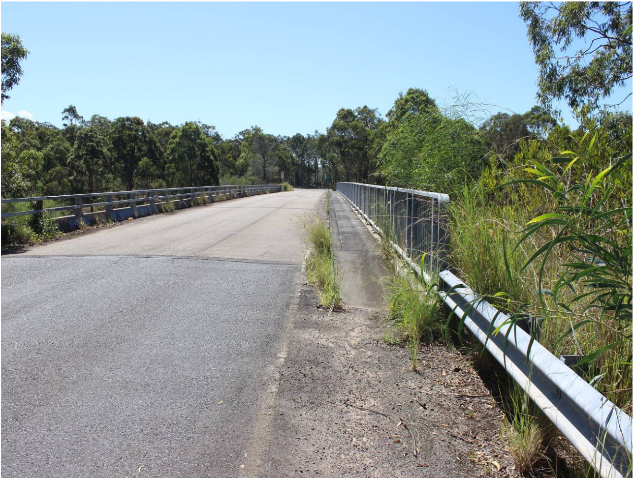
Photograph 7 – Overpass footway adjacent to the site
