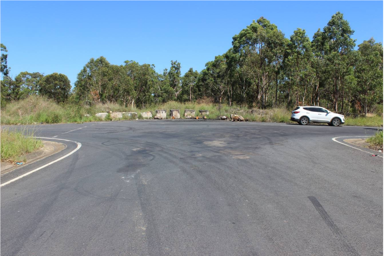
Photograph 1 – Site south of Motorway Link southern ramp / overpass road intersection
