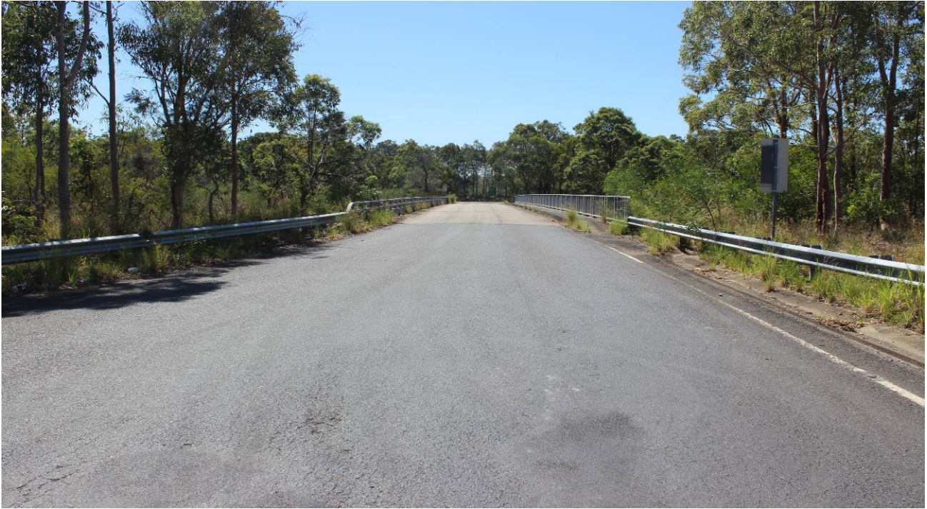
Photograph 5 – Motorway Link Overpass Bridge at Toohey's Road adjacent to the site
