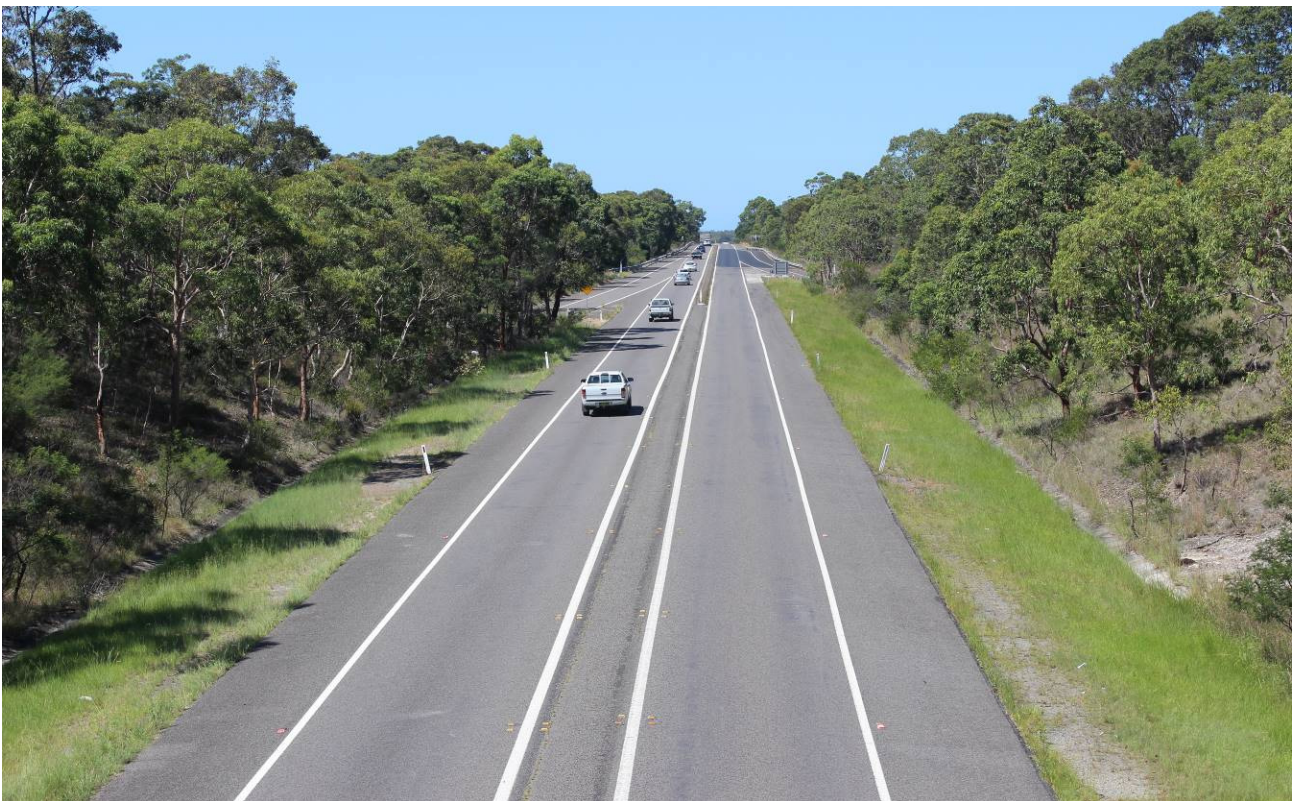
Photograph 3 – Motorway Link east of the overpass bridge
