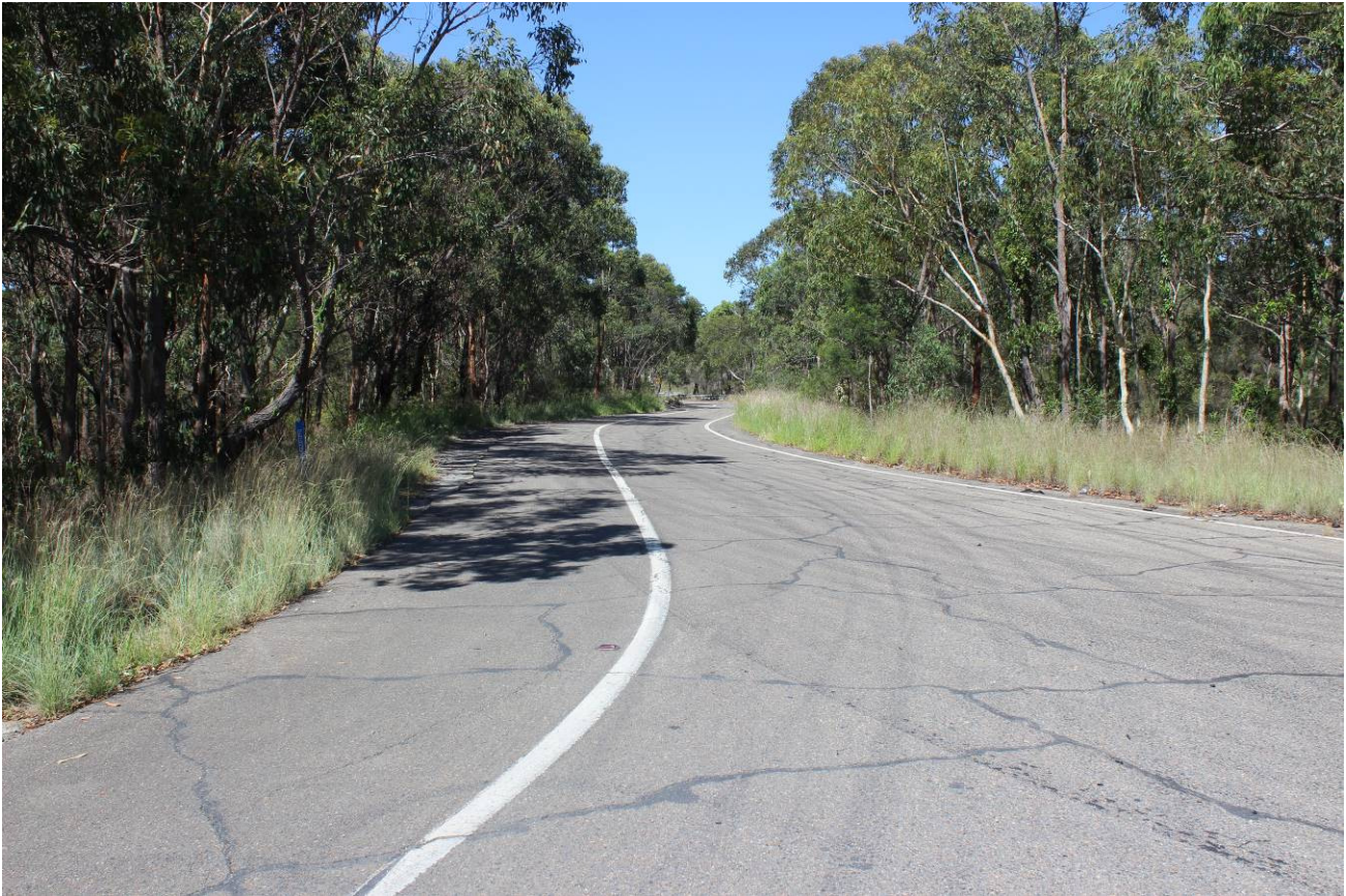
Photograph 4 – Motorway Link eastbound on ramp from Toohey's Road near the site
