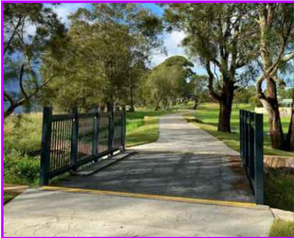
SMALL COMPOSITE BRIDGE SOURCE: CENTRAL COAST COUNCIL
