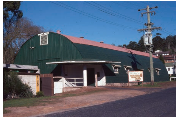
Public toilet block was built in 1979
