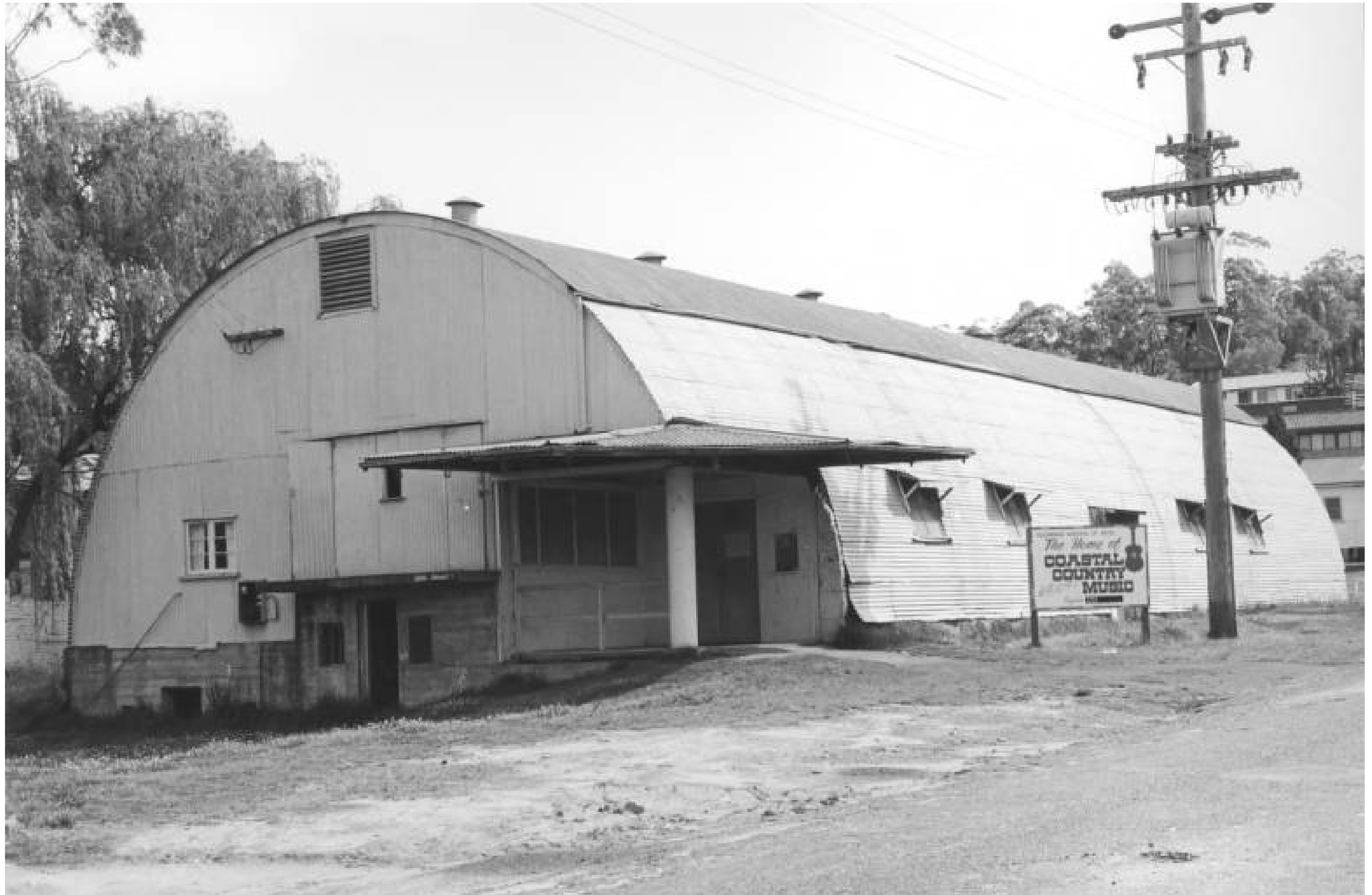
THIRD SCHOOL OF ARTS BUILDING, OURIMBAH - 1978
