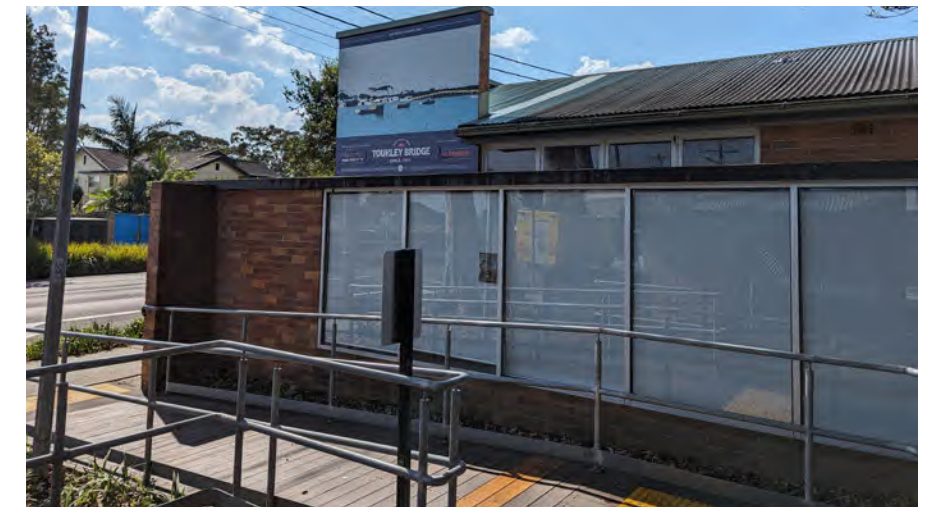
Hall canopy enclosed and entry from street blocked
