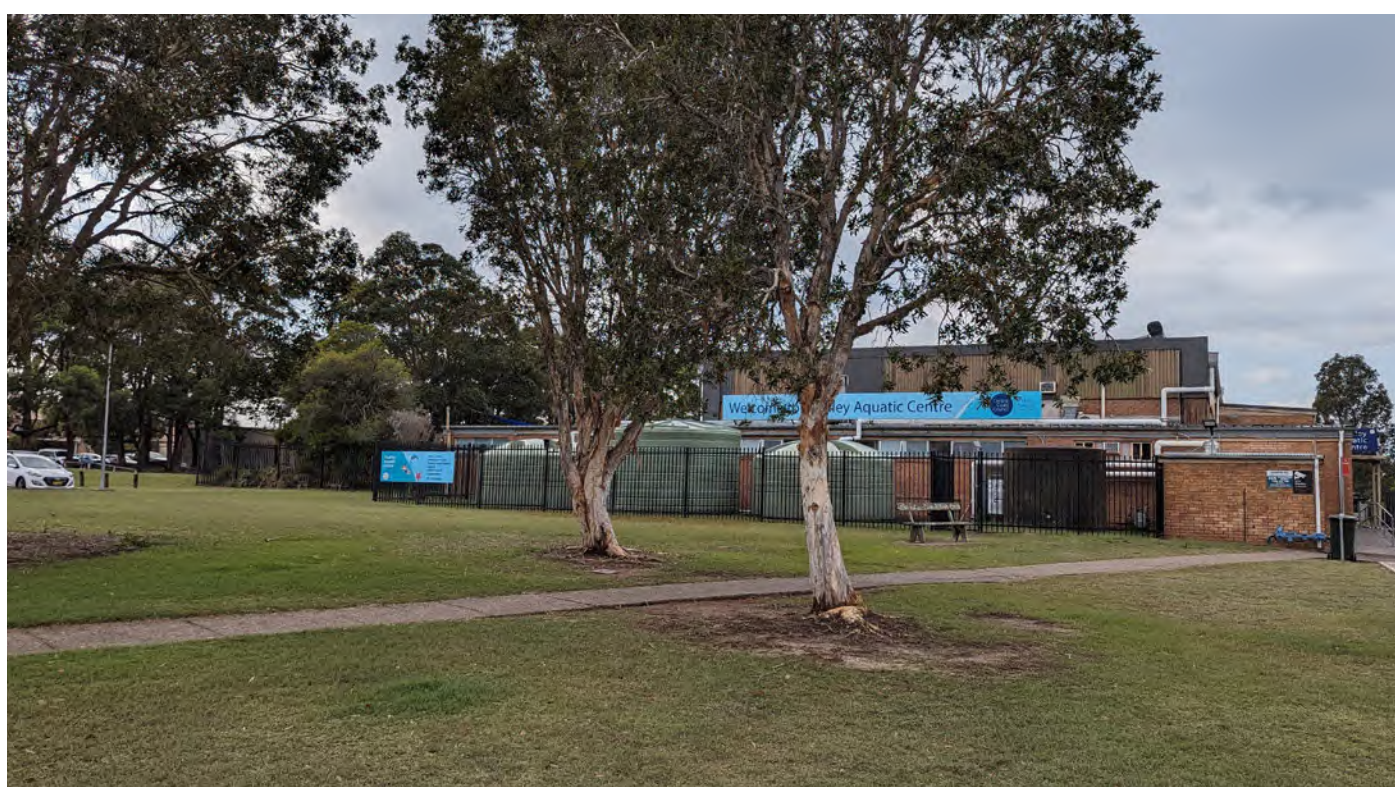
Footpath from western car park to aquatic centre entrance
