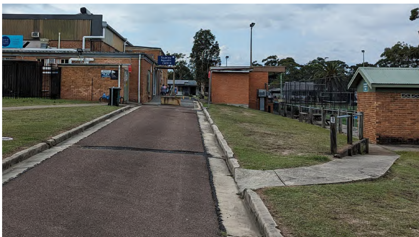
Existing access road
