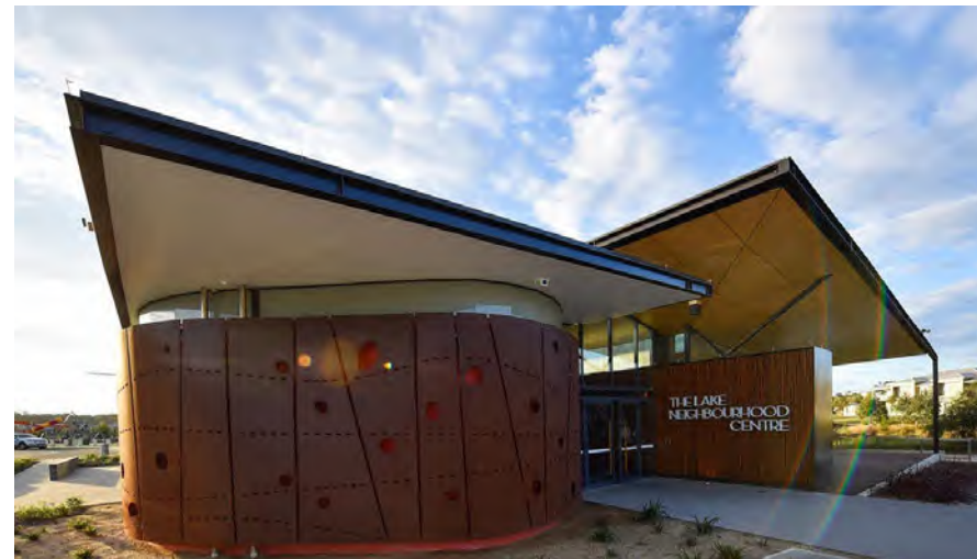
The Lake Neighbourhood Centre by Brewster Hjorth Architects
