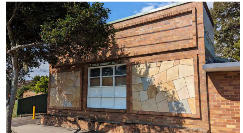
Historic hall facade
