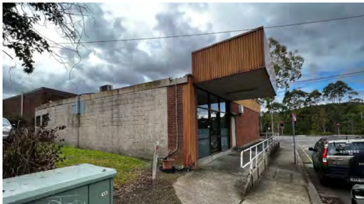
Ramp access to shops
