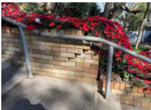
Figure 3.29 Stair landing showing metal handrail, cracked and bulging brick wall.
