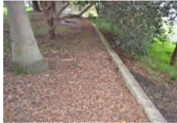
Figure 3.7 The buckled brick retaining edge at the top of the Memorial Park's western slopes.
