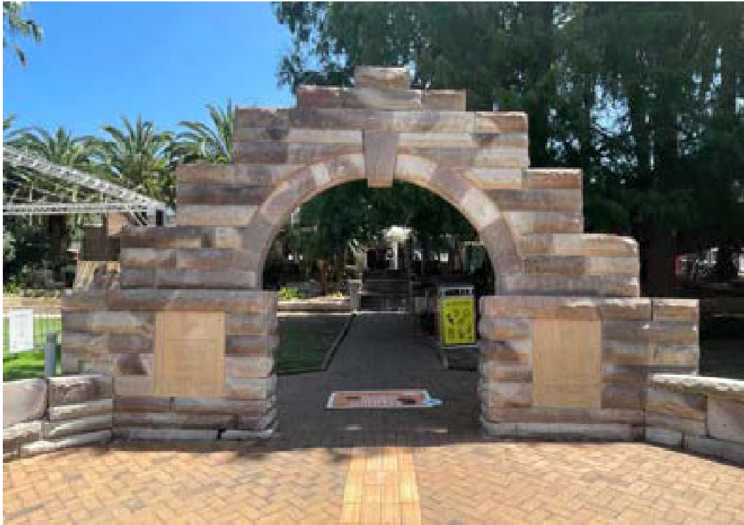
Figure 64: View of the eastern (front) elevation of the sandstone arch.
