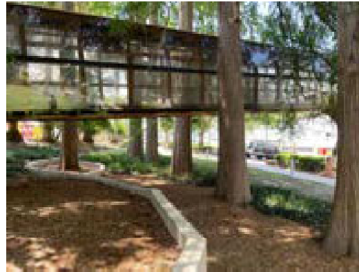
Figure 63: View of the footbridge from the park facing northeast.
