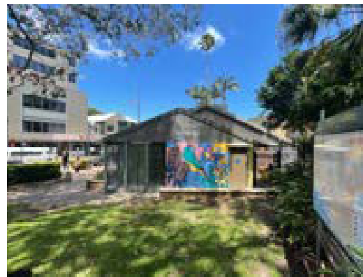
Figure 59: View of the northern wall facing south.
