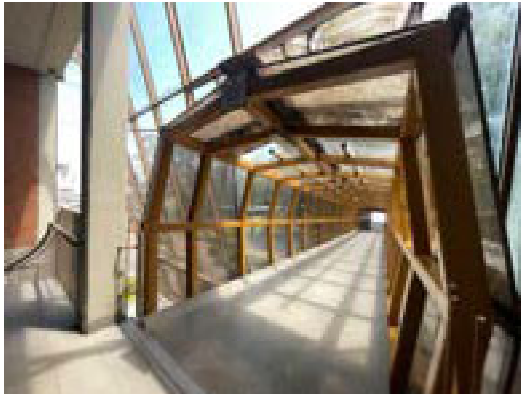
Figure 62: View of footbridge from the Gateway Centre facing west.
