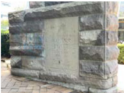
Figure 67: View of the stone panels in the base walls of the arch.
