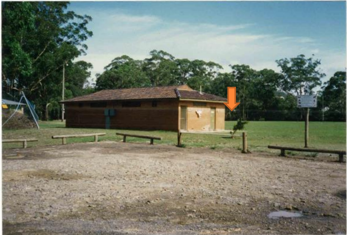
Figure ES3: Gavenlock Oval Flood level mark 3 bricks under bottom of window – February 1992
