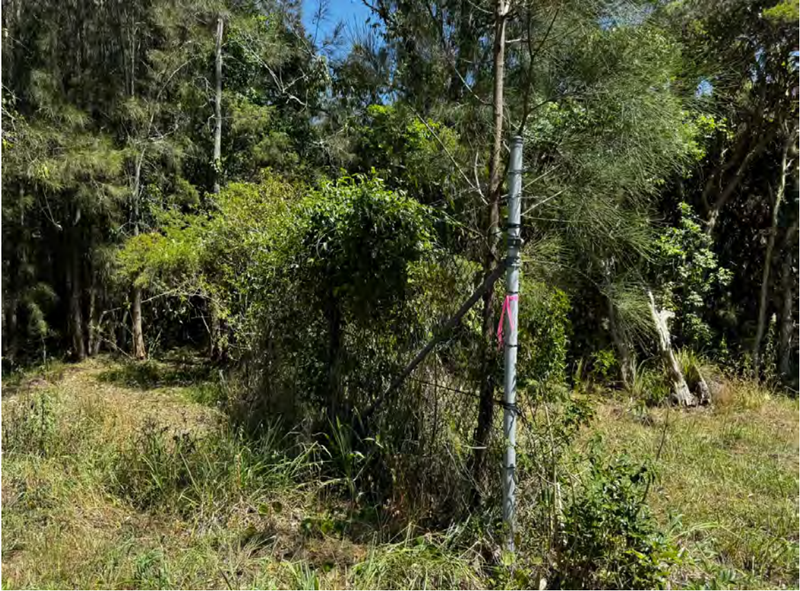
Photograph 5: Existing cyclone mesh fencing along the southern perimeter of the site
