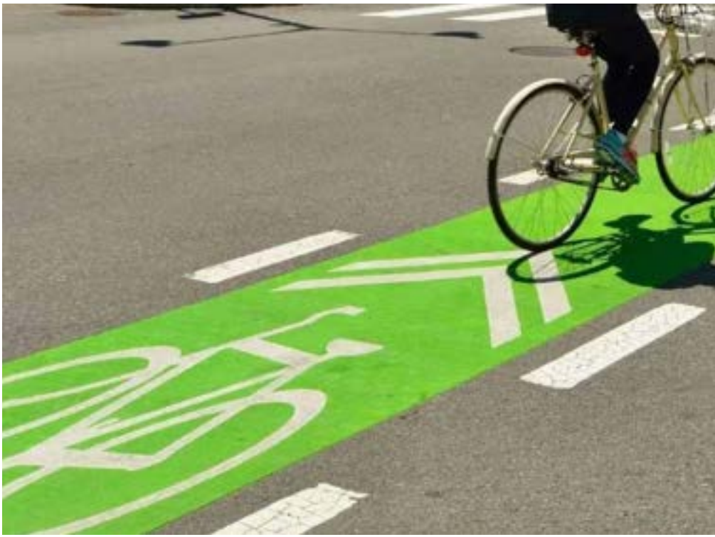
Cycle Hazard Markings
