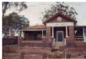
Former Court House
