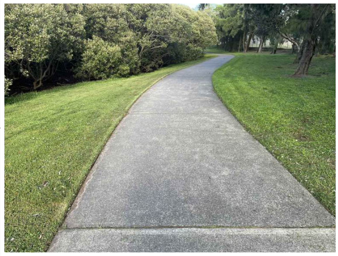
TYPICAL AT GRADE CONCRETE PATH
