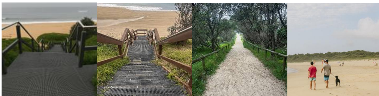
Fibre reinforced polymer frame and tread
