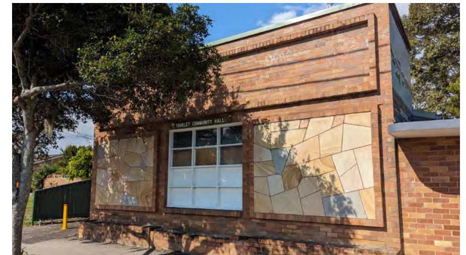
Historic hall facade
