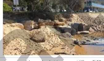
Stormwater scour and damaged pedestrian access at Killcare SLSC
