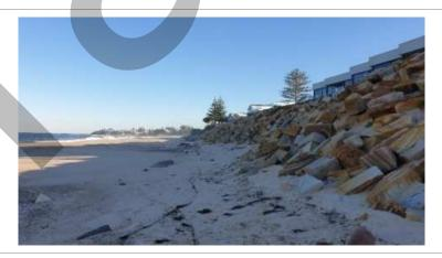
Unauthorised coastal protection works across the LGA (example shown at The Entrance North); works subsequently failed and slumped to the bottom of the slope in a storm event in May 2025
