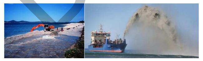
Figure 4-5: Examples of Sand Nourishment. Left: Jimmys Beach NSW. Right: "Rainbowing" – dredge pumping nourishment sand from offshore into the active beach zone (NSW Reconstruction Authority State Disaster Mitigation Plan, 2023)
