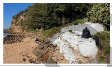
Ad-hoc coastal protection works at MacMasters Beach SLSC; works not engineered to provide protection against slope instability or beach erosion
