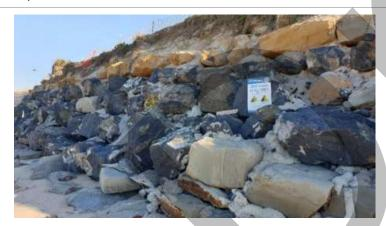
Erosion and undermining of seawall at The Entrance channel
