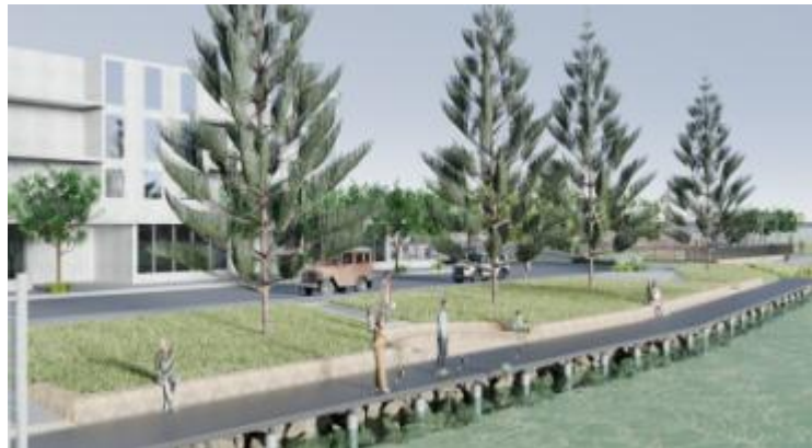
Figure 2 shows a continuous 3.4m wide foreshore platform for shared pedestrian and fishing access boardwalk along the foreshore.
