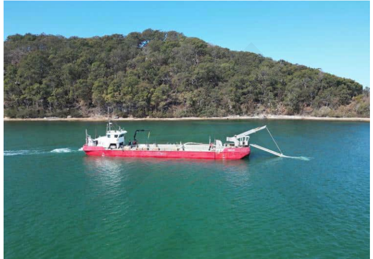
Figure 2-38 Dredging in the Ettalong Channel in 2025 (TfNSW, 2025)
