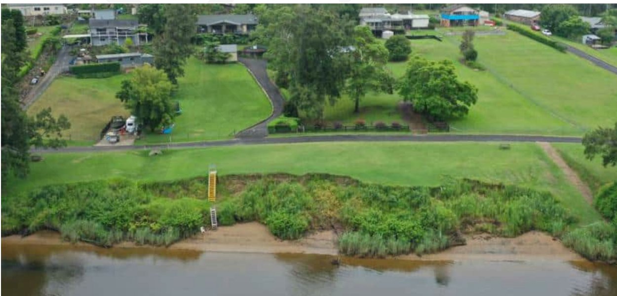
Figure 3-9 Bank erosion at Cumberland Reach (Alluvium, 2022b)
