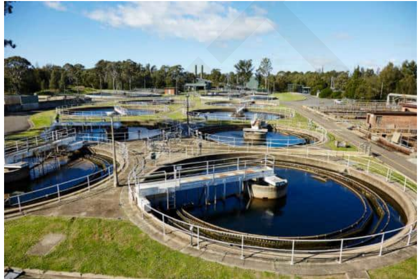
Figure 3-18 St Marys WRRF (source: Sydney Water)
