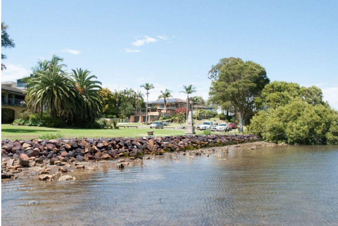
New Foreshore Protection Works Example
