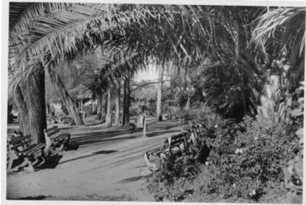
Figure 27: View of facing south towards the former rotunda structure, c1960. [Source: Central Coast Library Service]
