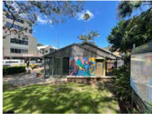
Figure 55: View of Burns Place facing south towards the bathrooms.
