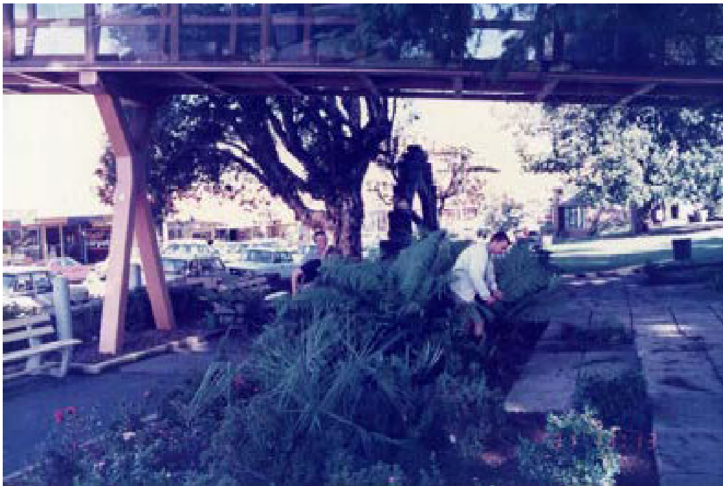
Figure 36: View of the underside of the pedestrian footbridge, c1985-1986, facing south. [Source: Central Coast Library Service]
