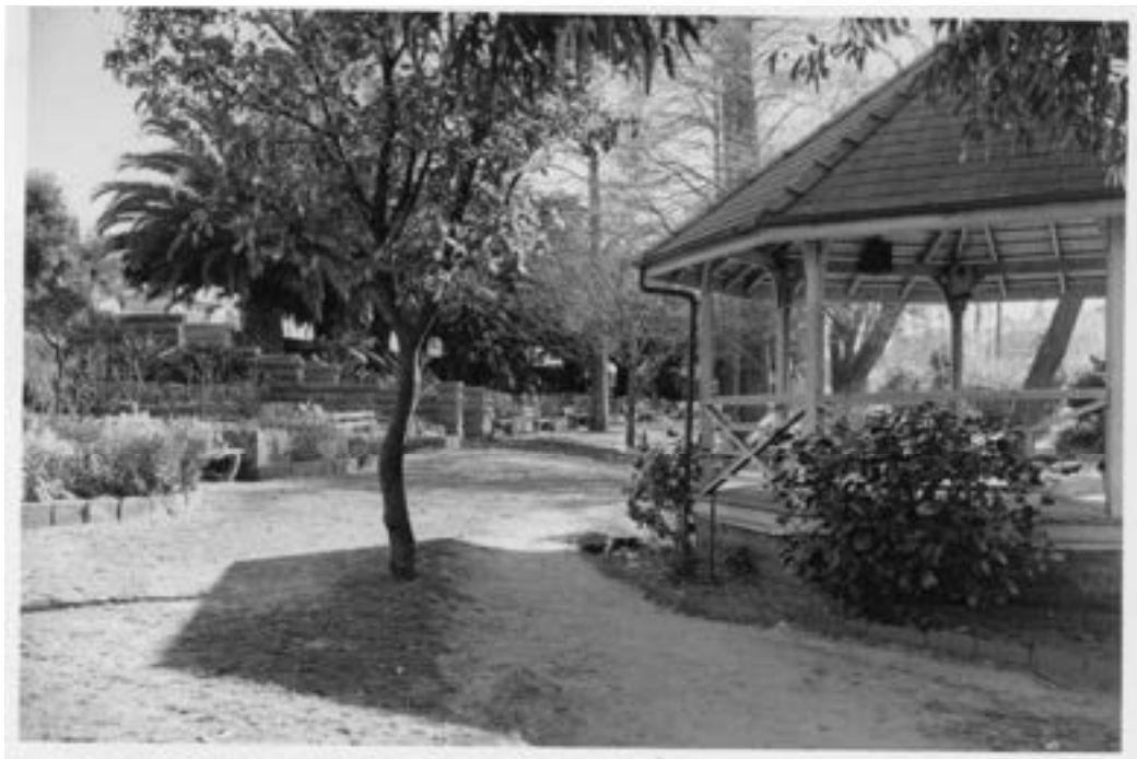
Figure 26: View of the former rotunda structure facing north towards the stairs to Gosford Railway Station (left of frame), c1960. [Source: Central Coast Library Service]
