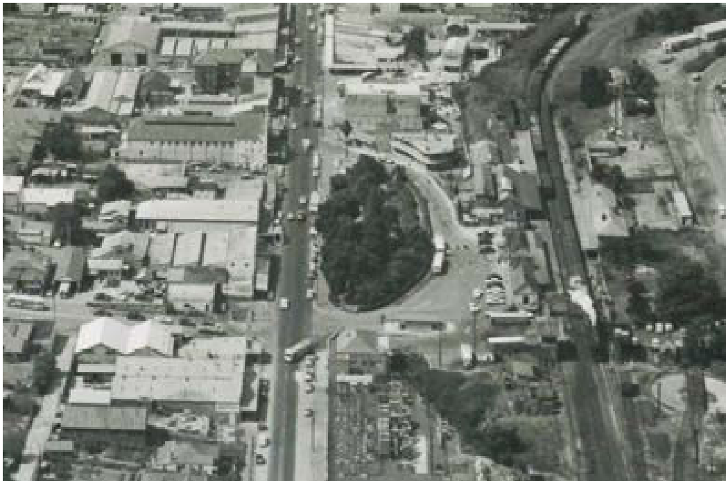
Figure 16: Aerial photograph of Burns Place, 1953. [Source: Photograph by Franklyn Wainman of Avion Views, Cooranbong NSW.]
