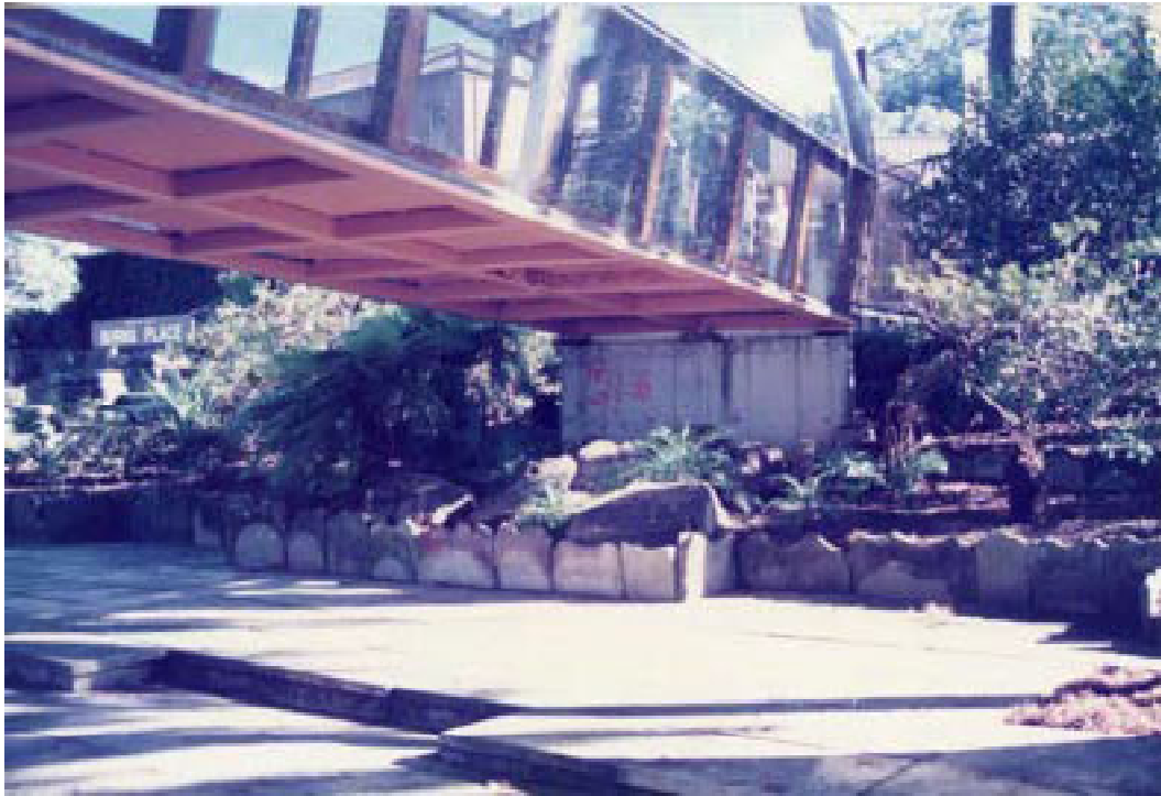
Figure 35: View the underside of the newly built pedestrian footbridge c1985-1986. [Source: Central Coast Library Service]
