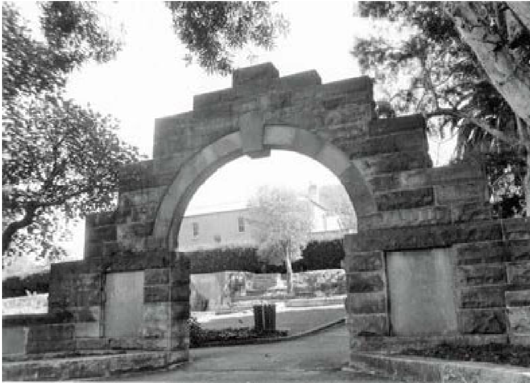
Figure 37: View of the sandstone arch facing west towards the former station masters dwelling. [Source: Central Coast Library Service]
