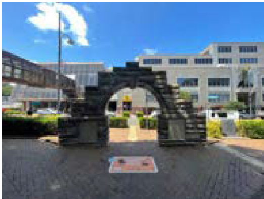
Figure 65: View of the rear elevation of the stone arch facing east.
